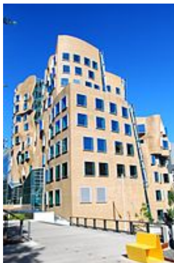
Dr Chau Chak Wing Building in Sydney, Australia (2014)
