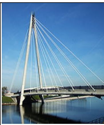
Marine Way Bridge
