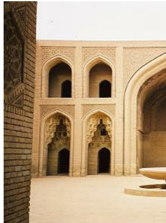
Figure 3: The building of a library in present day Baghdad, named after Ibn al-Bayhaqi, belongs to the collection of photographs taken by Nabil al-Tikriti, a member of the Islamic Civilizations at the University of Chicago to document damage to libraries in Iraq. It accompanies his report: Iraq Manuscript Collections , Arcadia Publishing, 2003.
